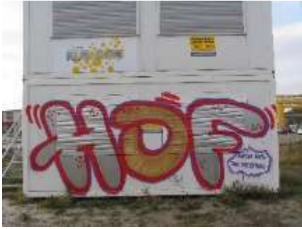
Container + window/blind + sign (Item: HDF)
