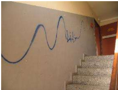
Closed interior + wall + staircase (Item: DiAS)
