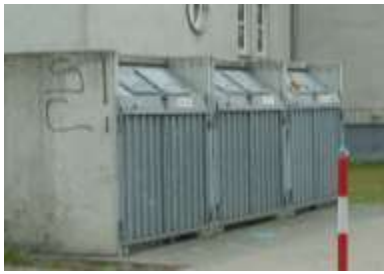
Waste/disposal containers + Wall (Item: SC!)
