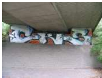
Column/Pillar/Support + Bridge + Wall (Item: CKS)
