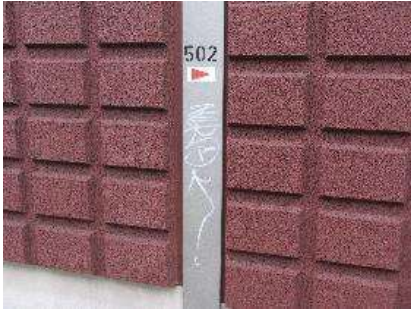
Noise barrier (Item: NeRO1)
