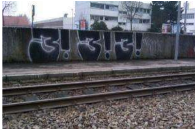
Track line + wall (Item: 3!)
