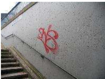
Underpass + wall + stairs (Item: SWS)
