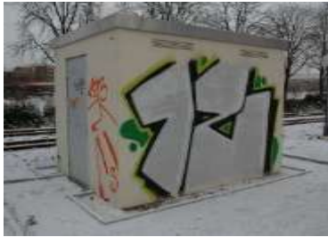
Railway line + wall (Item: 12)
