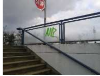
Railing/handrail + Stairs (Item: ANe)
